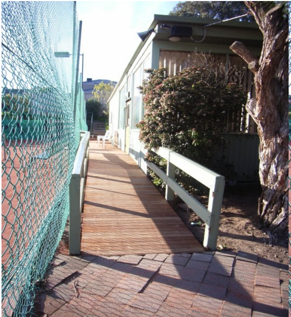
New ramp on western side
