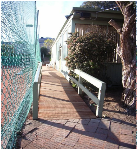
New ramp on western side
