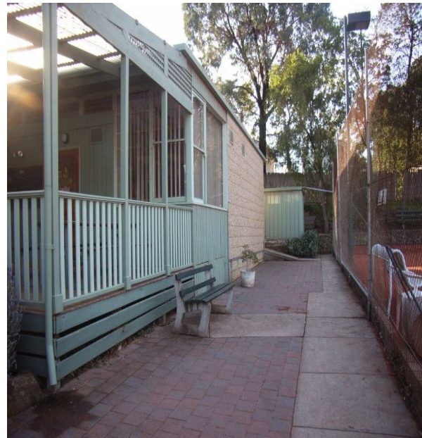
Site for three water tanks
